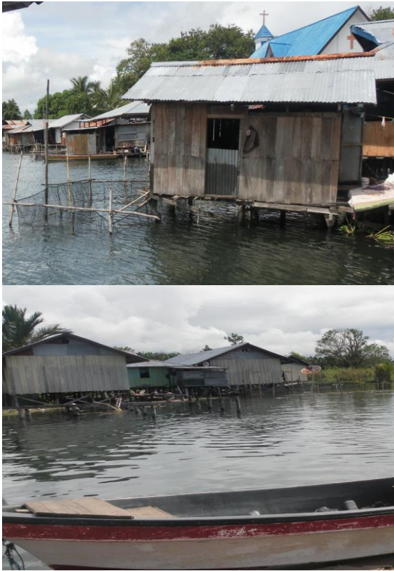
Figure 4. Inhabitants' Houses Built above Water
